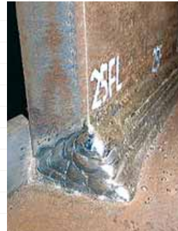
● Example of horizontal process (bead external view)
