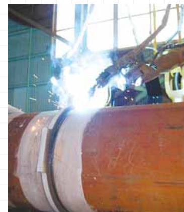
Round pipe 2-ARC welding
